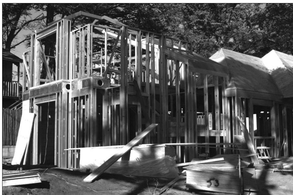
With its old-world exterior (above), the new home at Carmelo and 14th looks as if it's been there a long, long time. But in 2002, its ultra-modern, and termite-proof, framing was evident (below). Not only the posts and beams, but all the studs, are steel.
