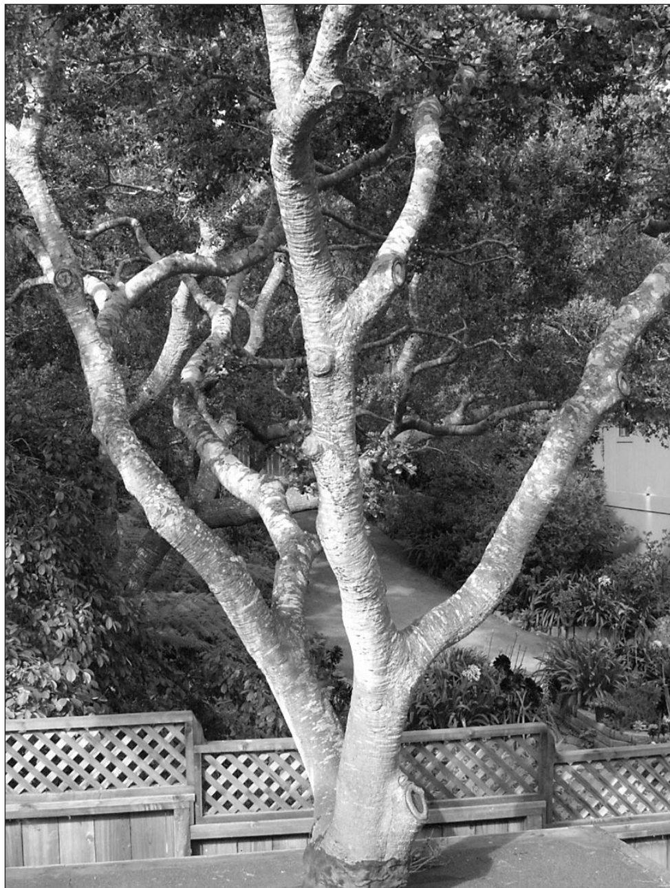
Viewed from above, the oak at Greg Baird's house seems to spring from the roof but is actually rooted in the ground, about 10 feet below. Flashing is tarred right to the tree to prevent leaks.
